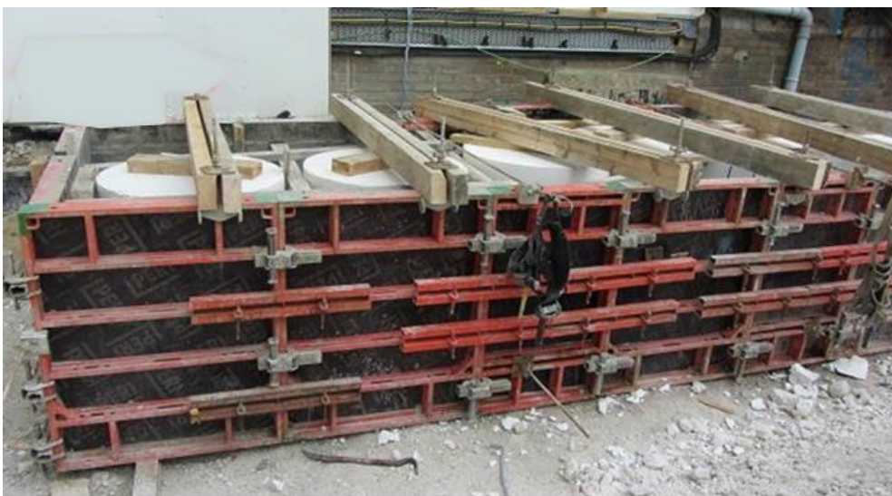
One of the piling frames with the polystyrene guides in place.
